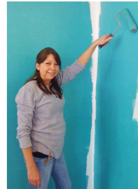
Store manager Danna Wall painted the walls.
